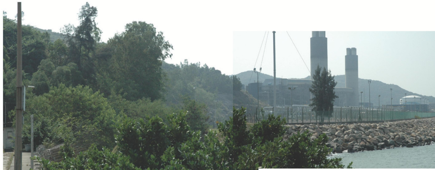
VSR7 - POWER STATION
